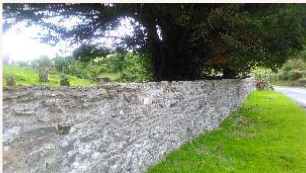
Dry-stone wall repairs coordinated by Hollywood Tidy Towns group.
