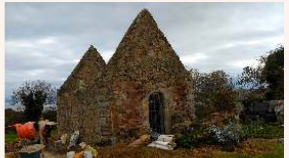
St. Crispins Church Greystones was repaired under the BHIS in 2014.
